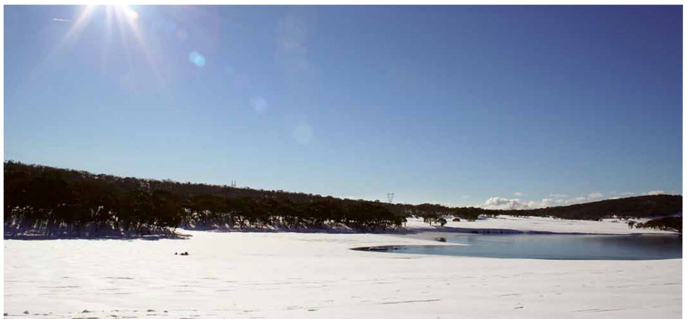
Three Mile Dam. Photo: Jo Caldwell
